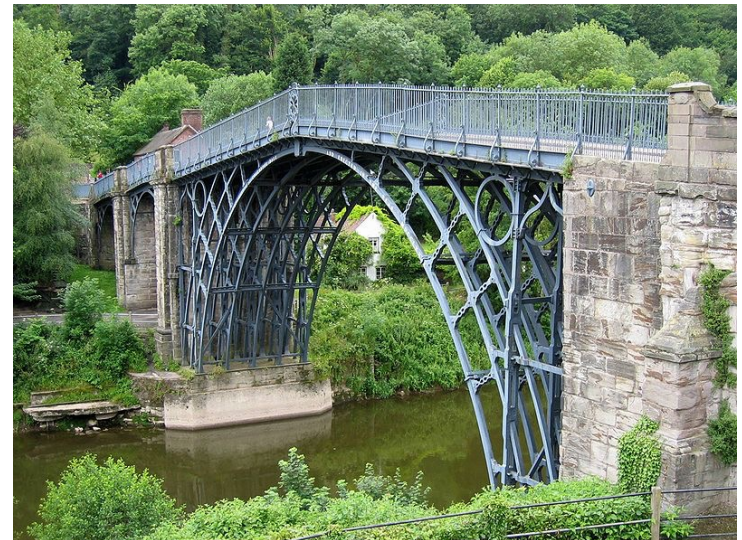
Iron Bridge, Shropshire. First bridge constructed from iron. Opened 1781.
